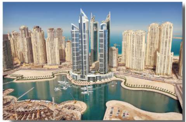
Bay Central Dubai-UAE
