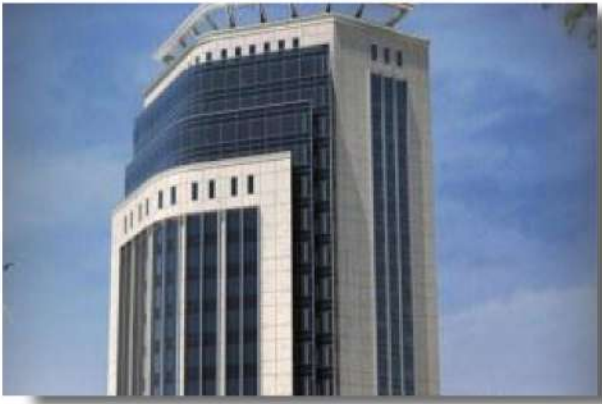
Al Baraha Tower Qatar
