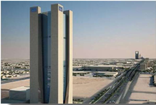
Al Rajhi Bank HQ, Riyadh Kingdom of Saudi Arabia
