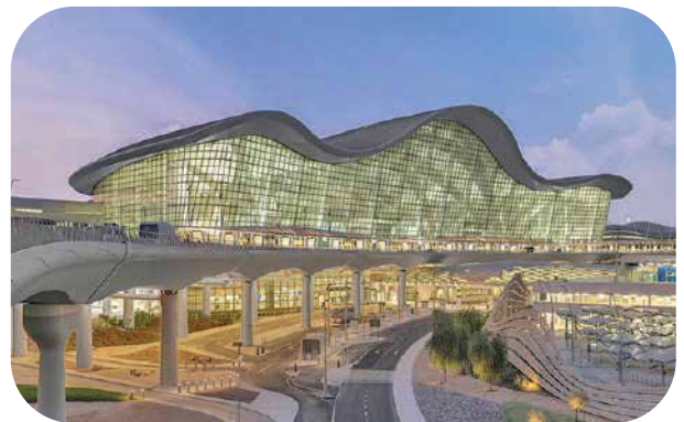
ABU DHABI AIRPORT, UAE
