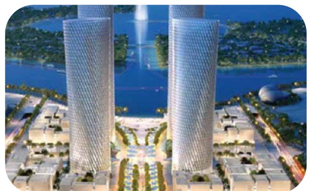
LUSAIL PLAZA TOWERS, QATAR
