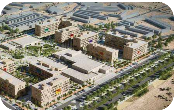
DAS ISLAND RESIDENTIAL DEVELOPMENT, ABU DHABI, UAE
