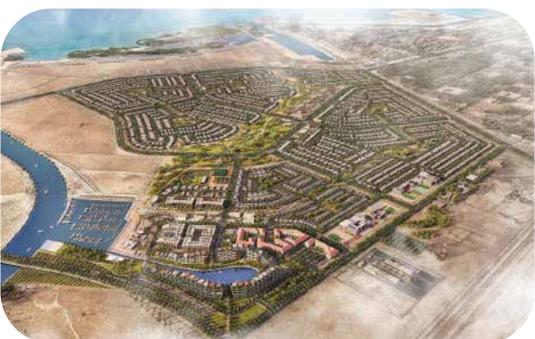
BALGHAIYAM DEVELOPMENT ABU DHABI, UAE
